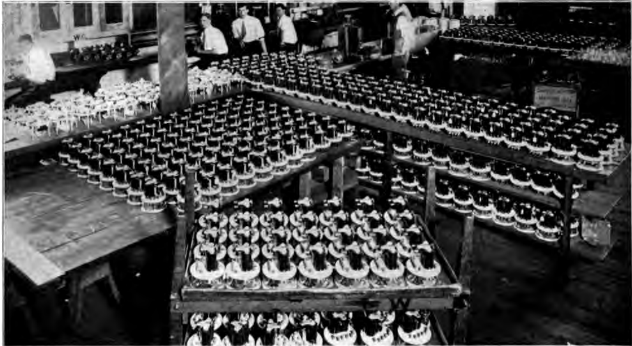
A Section of the Relay Department. Relays Ready for Test
